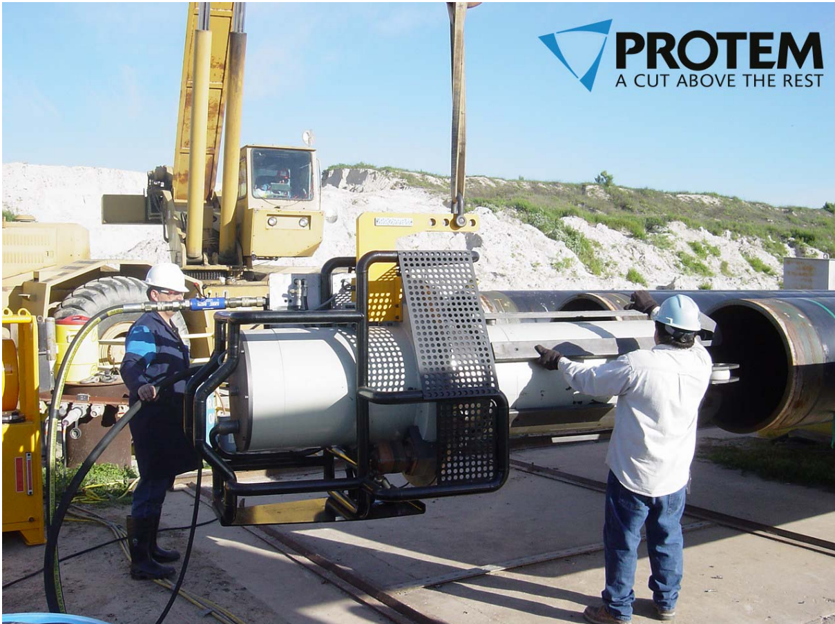
Figure 13 Welding preparation consisting in a J bevel for a pipeline laying. Use of a Pipe Facing Machine PROTEM US 620HSB
